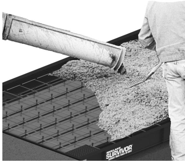
Figure 6-3. Pouring Concrete into Module
