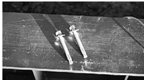
Figure 4-9. Anchor Bolts with Washers
