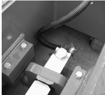
Figure 5-3. Load Cell Pocket Conduit Installed
