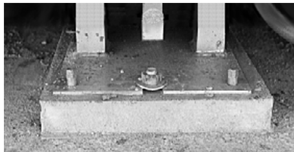
Figure 4-13. Completed Baseplate Grouting
