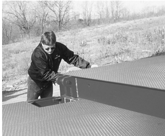
Figure 3-5. Module B Installation
