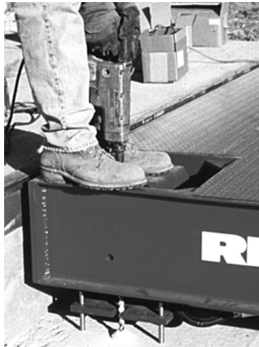
Figure 4-8. Drill Anchor Bolt Holes
