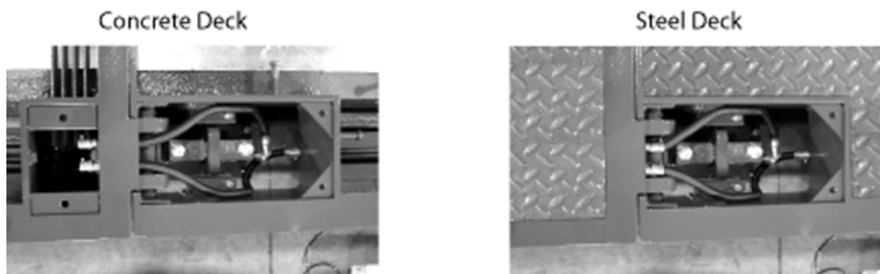
Figure 5-5. Conduit Connection Between Deck Modules
