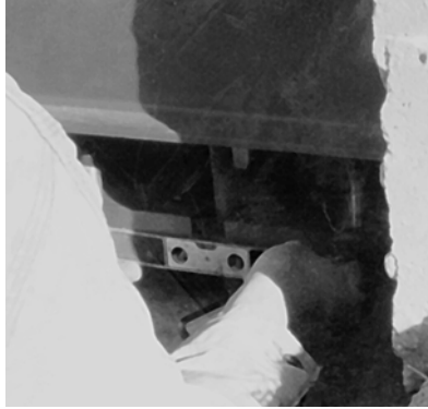
Figure 4-7. Recheck Link for Binding
