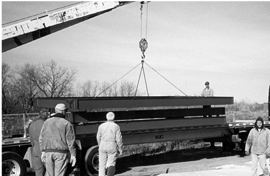
Figure 2-3. Lifting Deck Modules (Concrete Deck)
