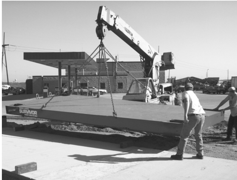
Figure 2-1. Lifting Deck Modules (Steel Deck)
