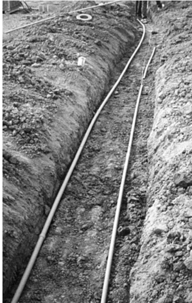
Figure 7-1. Conduit Run in Trench
